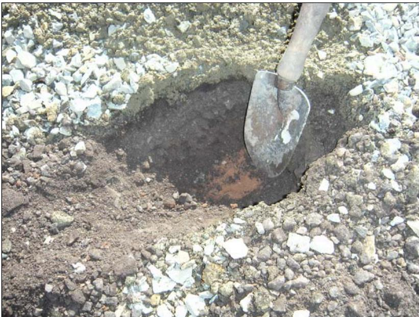
However, south of CR 42 (West side, near crest of hill) similar pits showed that a couple inches of base course were covering four inches of remaining asphalt, over what appears to be red clay from excavation at General Goodwin culverts. (This could be local soil.)
