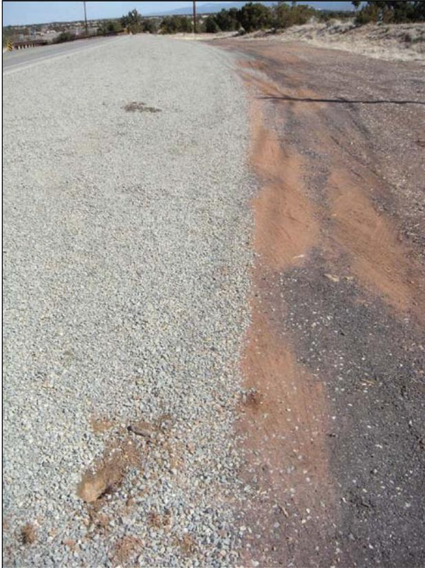
At NM 42 (LEFT), small pits dug at random locations into the new base course appear to show that the waste asphalt was removed (except for trace amounts) before base course was placed.
